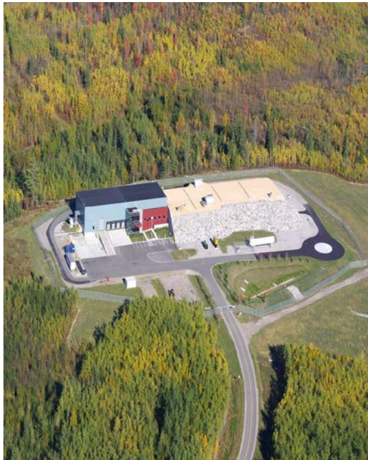
Figure 3: Far Detector Building in Ash River.
