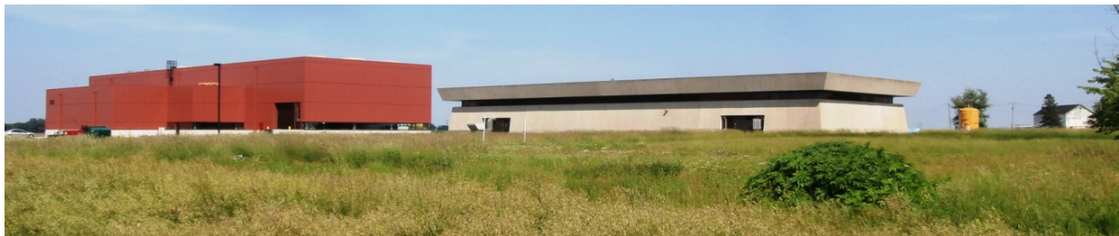
FIGURE 1. Photograph of the CMTF Building (left) and the NML Building (right)
