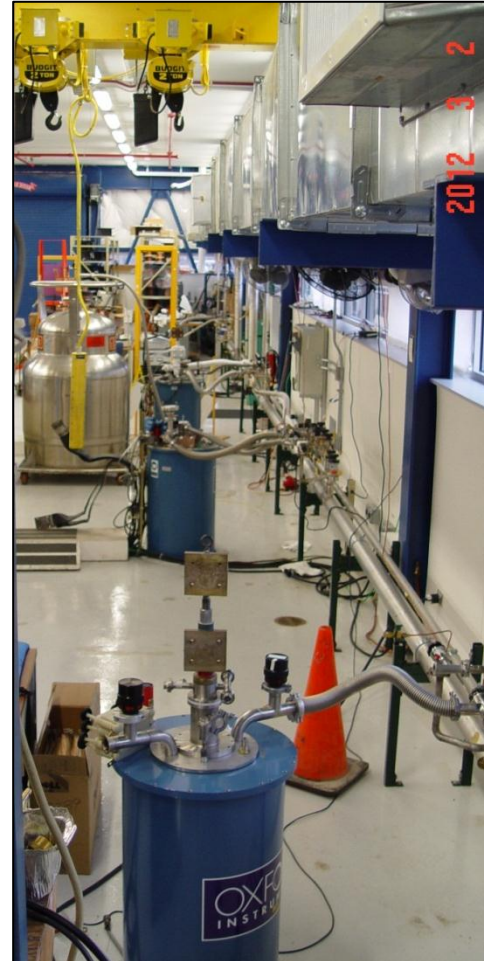
Fig. 5. Four cryostats with up to 15T/17 T background field, and with cold apertures between 64 mm and 147 mm are connected to new vent and vacuum systems.
