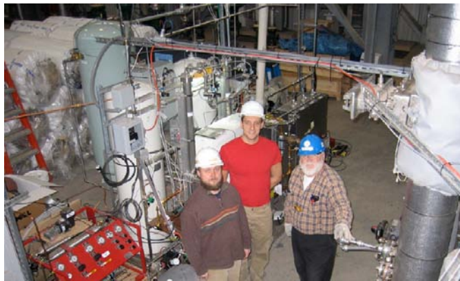
Figure 2. VPSA system in Cortez, CO.
