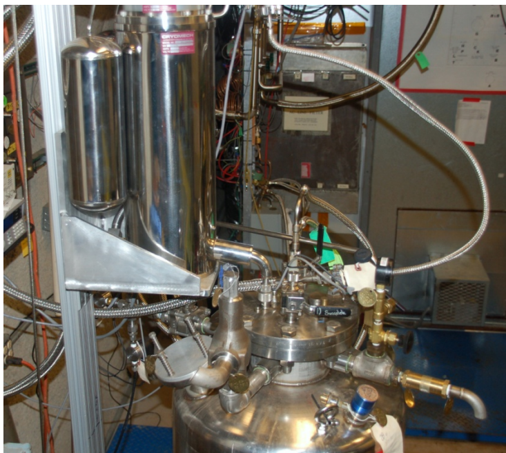
FIGURE 1. Cryomech PT15 re-liquefier installed in 120 liter external cold trap cryostat. Lifting bracket on left, cryocooler drain line in middle, cryostat lower center
