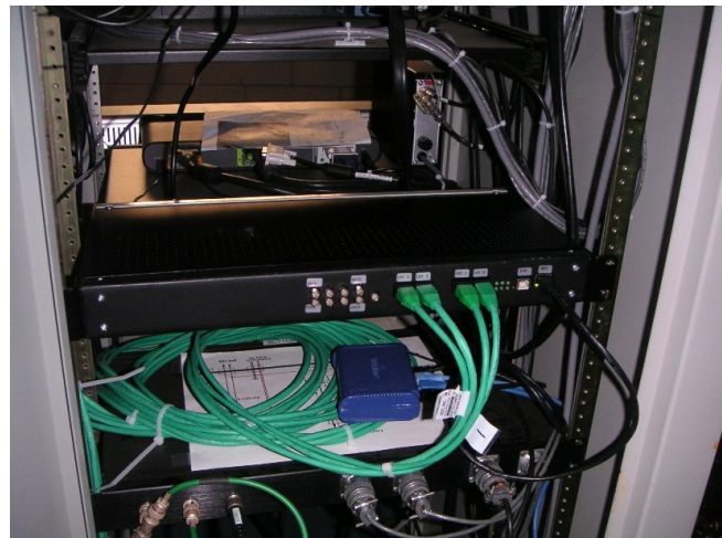
Fig. 3. Photograph of the controller installed for four liter test run at Fermilab. The green cables are the PMT links, the black is the Ethernet cable. The LEMO inputs are visible to the left of the PMT links.
