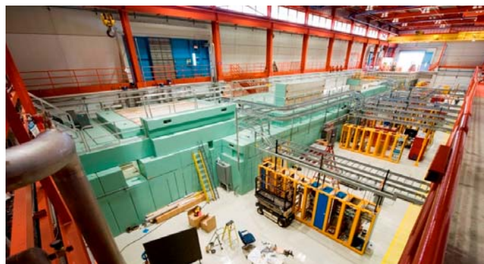
Figure 1: Current interior of NML, looking downstream from the injector end.
