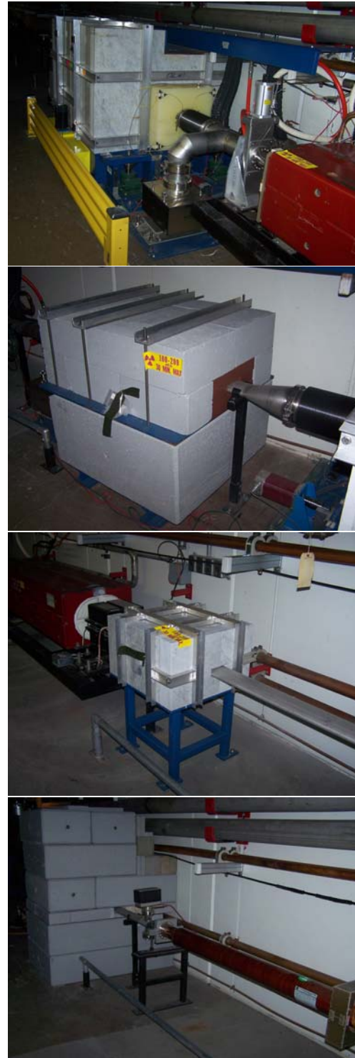
Figure 4: Examples of installed collimators: 20-Ton Secondary, steel and concrete mask (STCM), steel and marble mask (STMM) and the concrete wall are shown.
