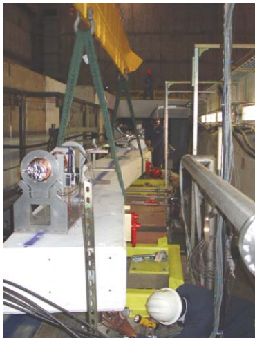
Figure 2: Installing the girder supporting the BPM3-5 triplet.
