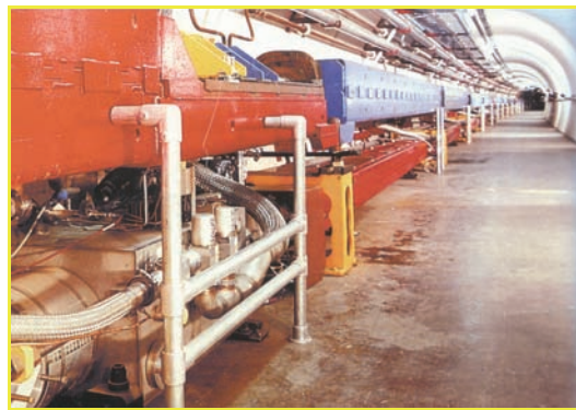
Picture 2. View of Tevatron tunnel
