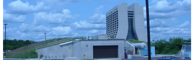
Figure 7: Picture of the MTA at the south end of the Fermilab linac.
